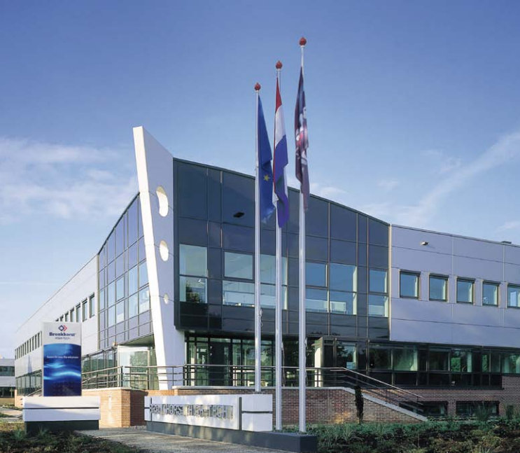
Bronkhorst High-Tech headquarters, The Netherlands
